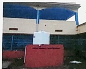
Rain Water Harvesting
