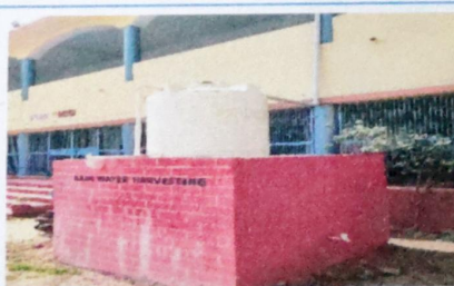
Rain Water Harvesting
